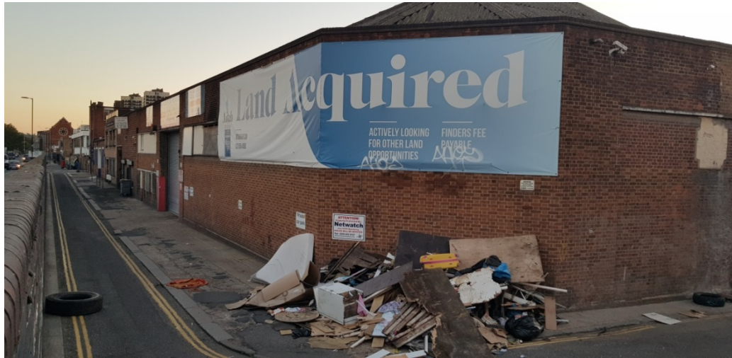
Figure 1: View of existing site at 134-140 Ilderton Road, Record Street (east side) and Ilderton Road
